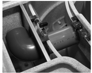
Figure 17.3 - By-pass in operation
